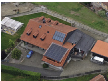
47 m 2 – 11.7 kWc 1691 Villarimboud
