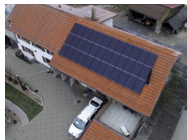
55 m 2 – 10.8 kWc 1691 Villarimboud
