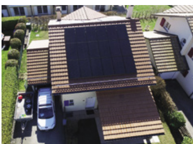
30 m 2 – 5.4 kWc 1186 Essertines-sur-Rolle
